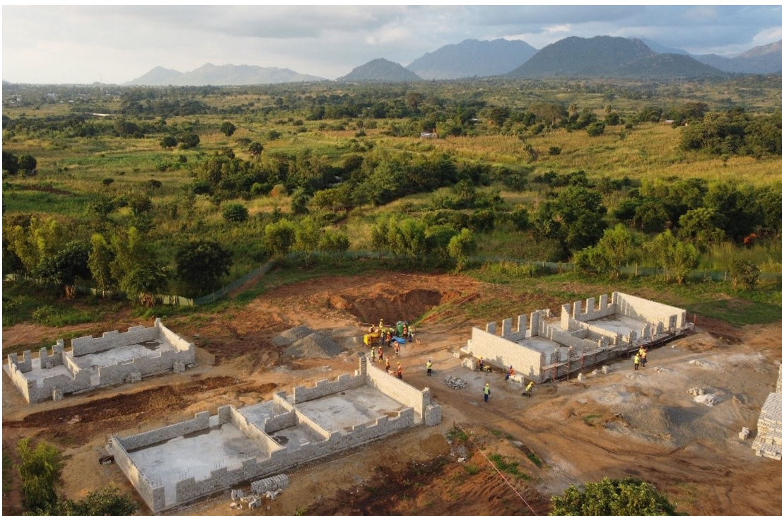
Construction of rural SEED community day secondary school.
